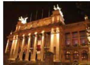
The museum's façade lighting has been replaced by a LED lighting solution by THORN. Individual areas of the façade are precisely illuminated. The entire façade lighting is controlled by a LUXMATE lighting management system. Compared to the former lighting system, this has led to an overall drop of 50% in energy consumption.
