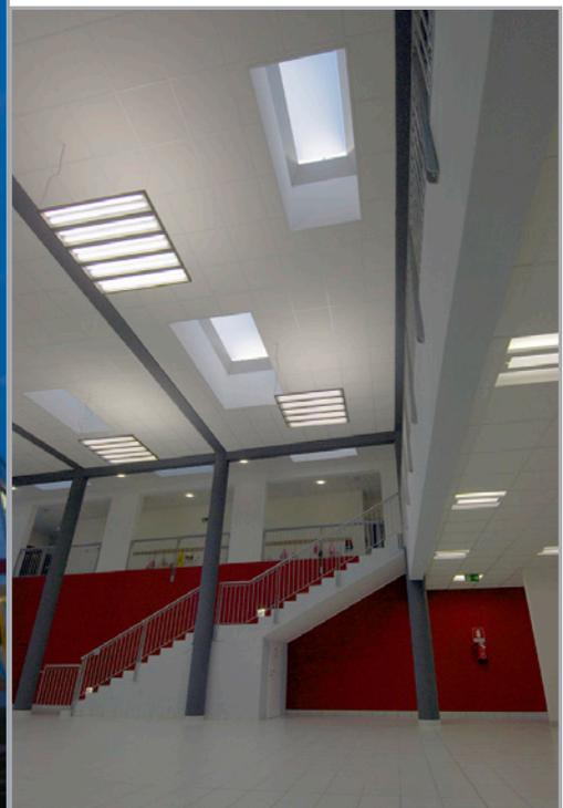
**Thorn: Primary School Vicentino (IT)** Through the intelligent use of natural light and an innovative lighting solution from Thorn, energy consumption at this primary school has been reduced by 70 percent. All luminaires are dimmable and controlled by a daylight-based SensaModular system.
