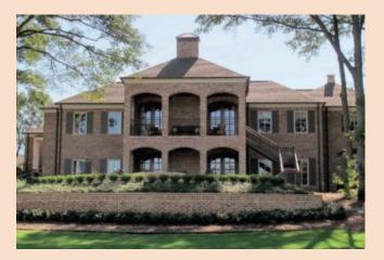
The "papercut brick" is an exclusive facing brick that looks like an old, hand-molded brick. Its name is derived from the production process. Recycled paper is rolled onto the pressed brick material, which is then wire-cut into individual
