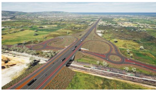
Extension of Tonkin Highway and widening of Thomas Road © Georgiou Group
