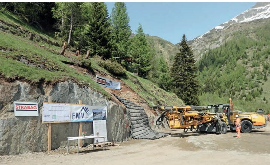
STRABAG AG is building a 14 MW run-of-the-river hydroelectric plant in the Swiss canton of Valais. The contract value of € 37 million (CHF 38 million) comprises the construction of the necessary tunnels, galleries and underground chambers. The tunnels and galleries will be excavated in the Aarmassif of the Swiss Alps through boring and blasting. The plant is to be handed over to Valais utility company FMV SA by September 2017.
