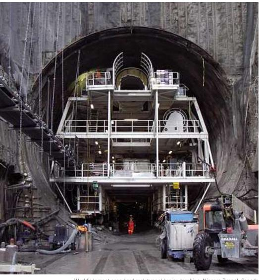
World's largest open hard rock tunnel boring machine, Niagara Tunnel, Canada
