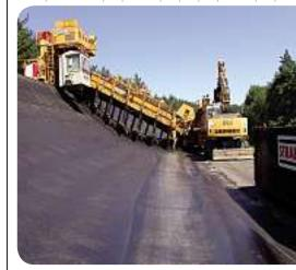
Asphalt finishing machine, Germany
