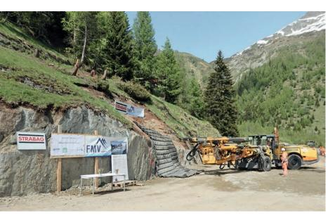
STRABAG AG is building a 14 MW run-of-the-river hydroelectric plant in the Swiss canton of Valais. The contract value of € 37 million (CHF 38 million) comprises the construction of the necessary tunnels, galleries and underground chambers. The tunnels and galleries will be excavated in the Aarmassif of the Swiss Alps through boring and blasting. The plant is to be handed over to Valais utility company FMV SA by September 2017.
