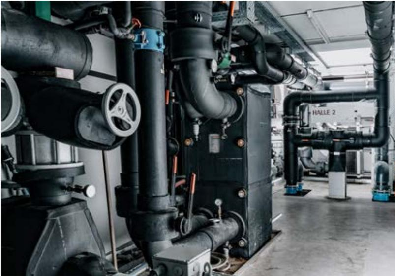
At the Ebensee plant, the injection moulding machines are cooled with groundwater.
