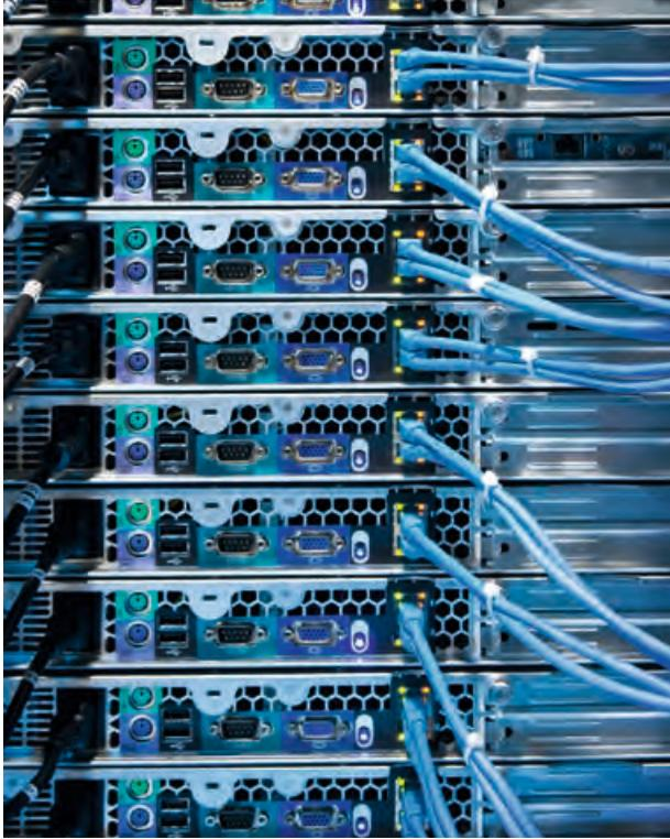
Modern high-performance data cables bring high-speed Internet into buildings. The coating of these data cables consists of ethylene and propylene.
