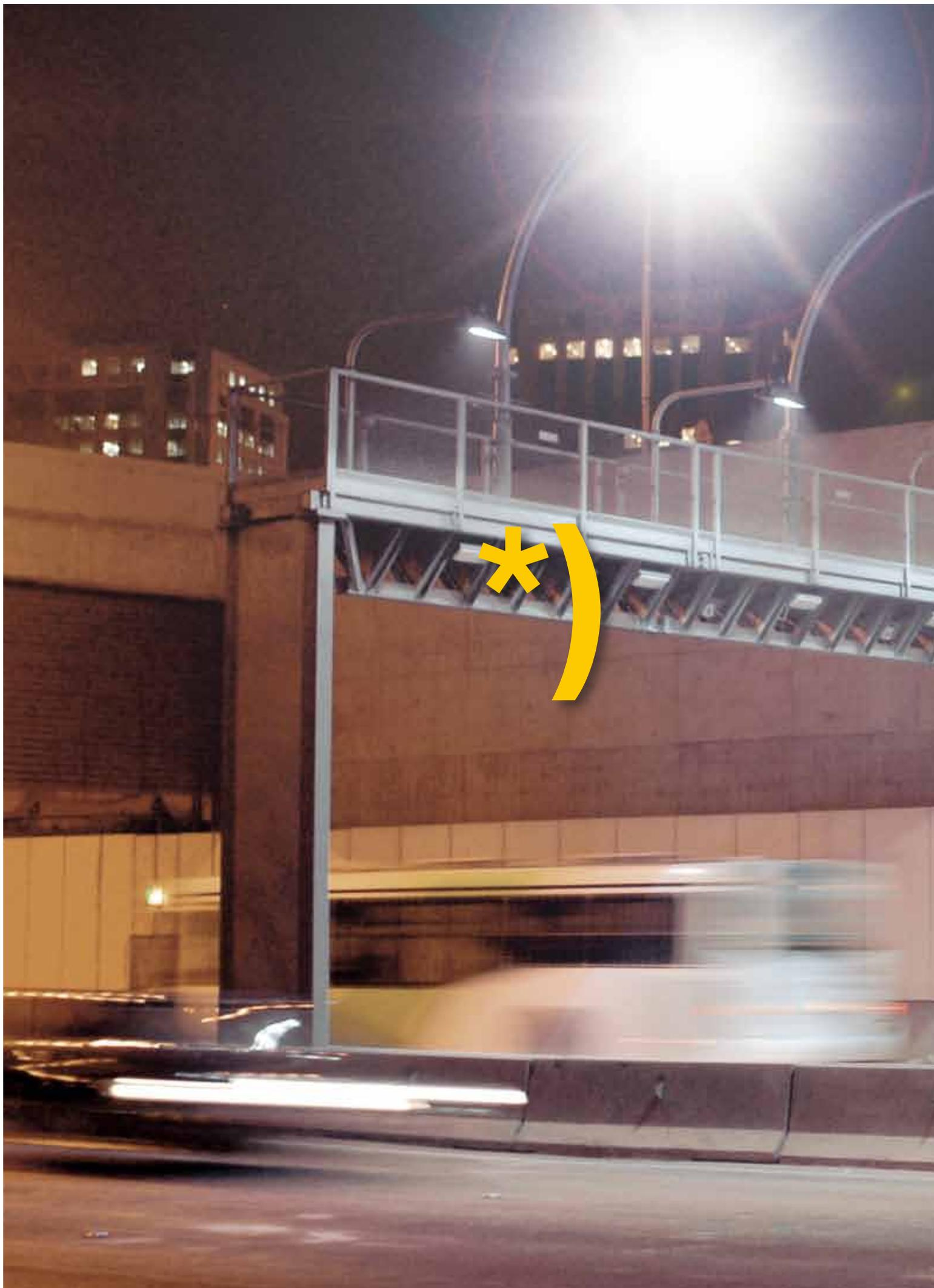
**\*) What you see here: Vehicles equipped with an on-board unit, enable electronic toll collection systems to charge fees fully automatically – without interfering at all with the traffic flow.**
