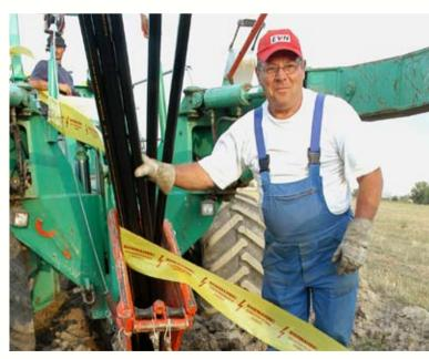
Underground cable laying using a special plough
