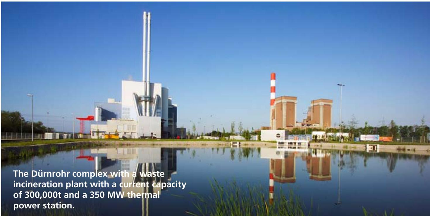
The Dürnrrohr complex with a waste incineration plant with a current capacity of 300,000t and a 350 MW thermal power station.
