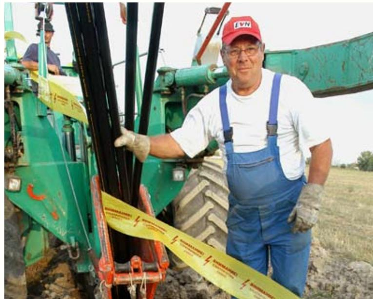
**Underground cable laying using a special plough**
