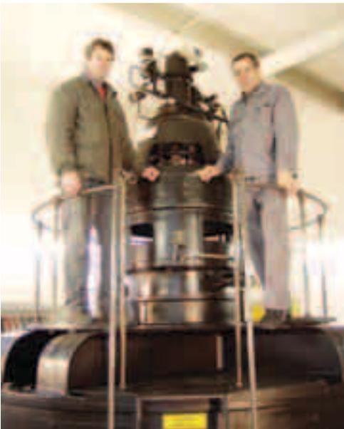
One of the most outstanding ideas for improvement is the grinding device designed by Rudolf Schoisengeier (r.) and Thomas Weiß (l.), which facilitates the on-the-spot repair of turbine bearings without disassembly.
