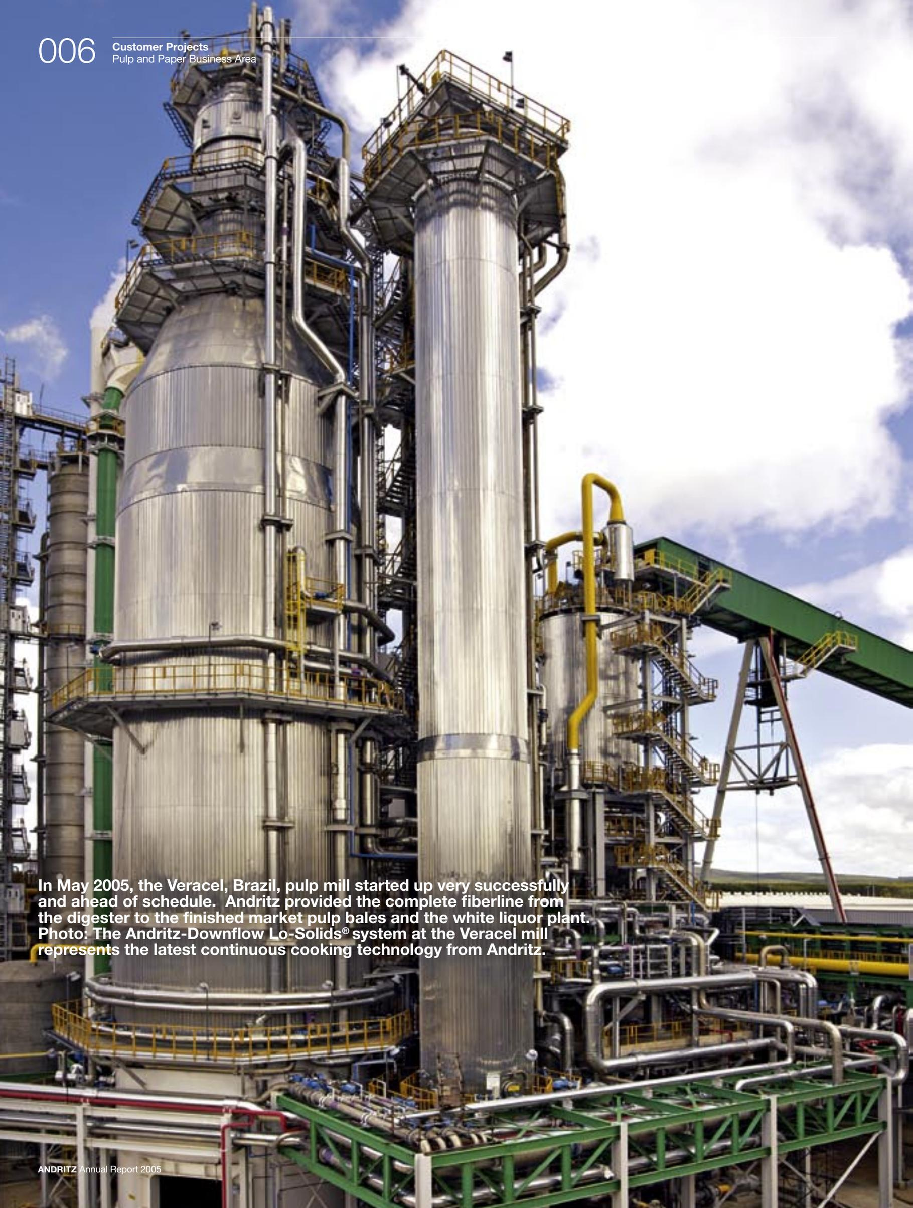
In May 2005, the Veracel, Brazil, pulp mill started up very successfully and ahead of schedule. Andritz provided the complete fiberline from the digester to the finished market pulp bales and the white liquor plant. Photo: The Andritz-Downflow Lo-Solids® system at the Veracel mill represents the latest continuous cooking technology from Andritz.
