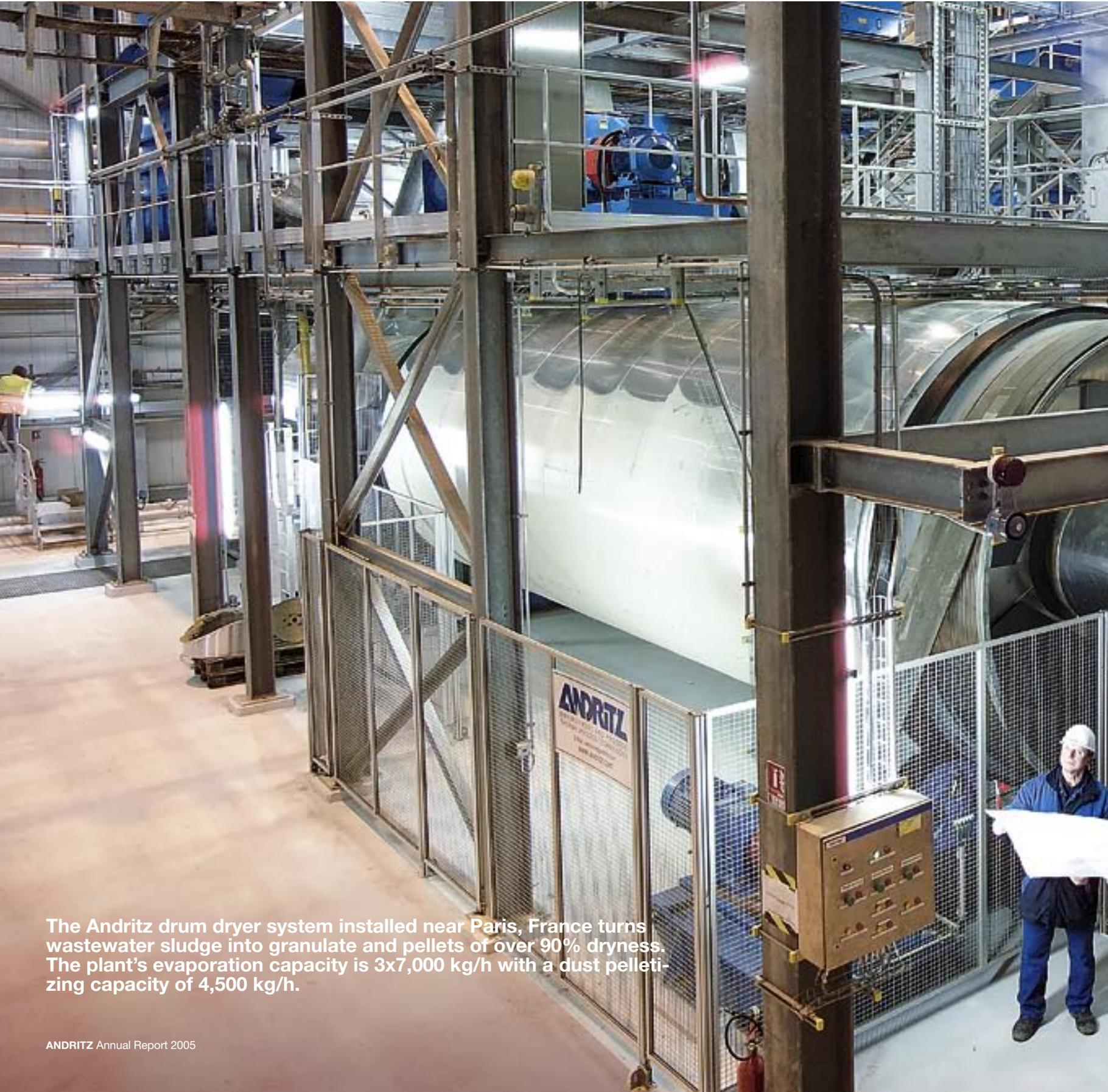
The Andritz drum dryer system installed near Paris, France turns wastewater sludge into granulate and pellets of over 90% dryness. The plant's evaporation capacity is 3x7,000 kg/h with a dust pelleting capacity of 4,500 kg/h.
