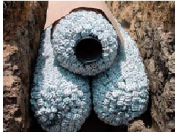
Drainage pipe with a covering made of EPS chips
