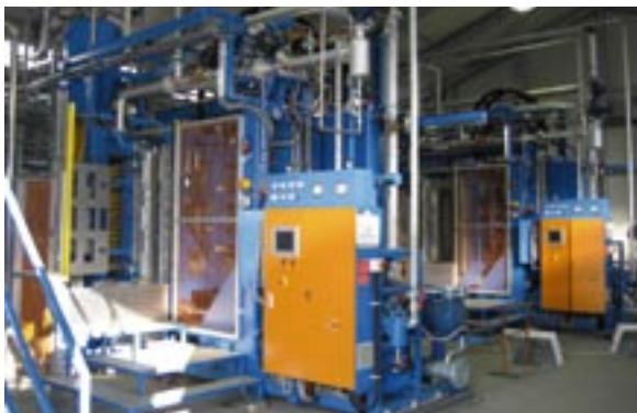
Interior view of 2 HS 1400 shape molding machines
