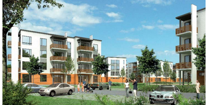
EE, Tallinn, Apartment building Haabersti
