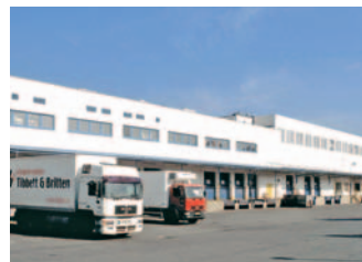
CZ-Prague Westpoint Distribution Park L N
