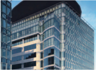
PL-Warsaw Crown Tower O N
